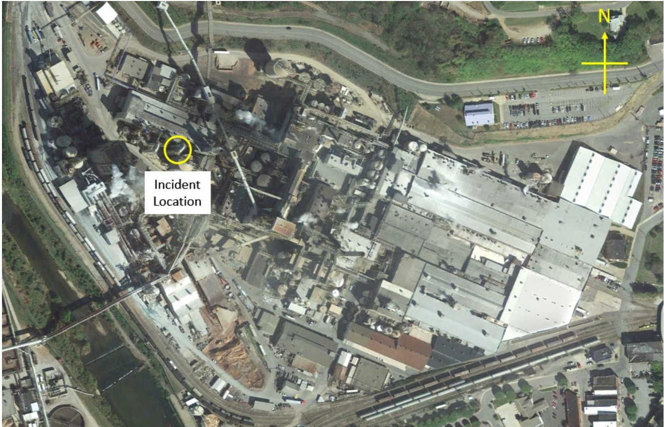
Figure 2. Overhead view of the Evergreen Packaging Canton Mill. (Credit: Google. Annotated by CSB.)
